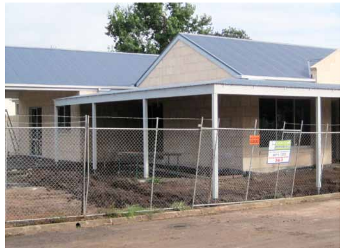
The new Merino Community Health Centre is rapidly taking shape.
